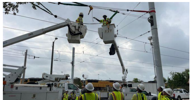
METRO employees work alongside contractors to replace an insulator.
