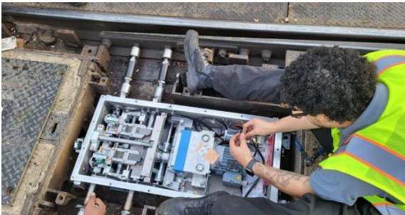
Crews work to replace a switch near Palm Center Transit Center.
